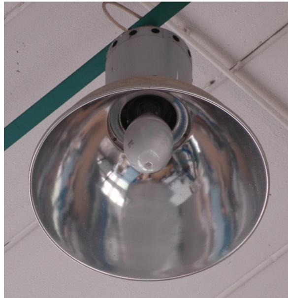
**Fig. 2.** A high-bay luminaire with a mercury vapor lamp.
